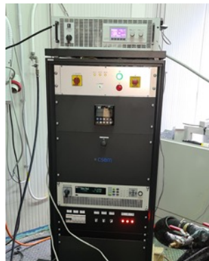
DC bus generator
